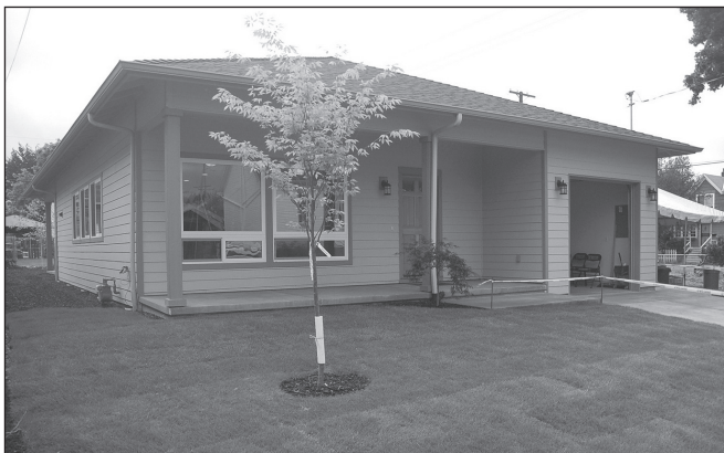
House built by Benson students completed in May 2012.
